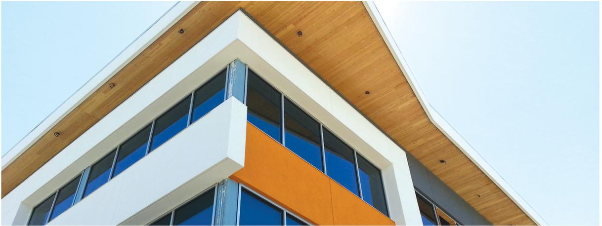
The CLT roof system forms an angled overhang along the entry side of the office building.
